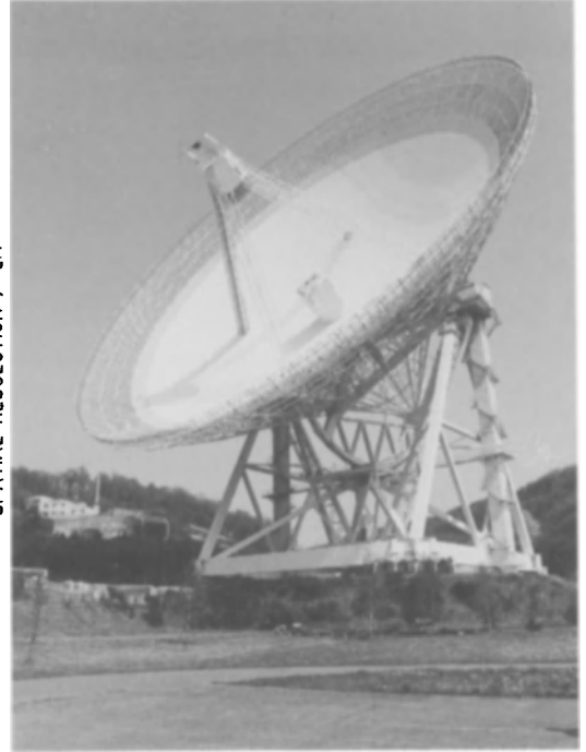
Fig. 14. The 100m radiotelescope, Effelsberg, Germany, the biggest VLB interferometer element routinely used for VLBI
